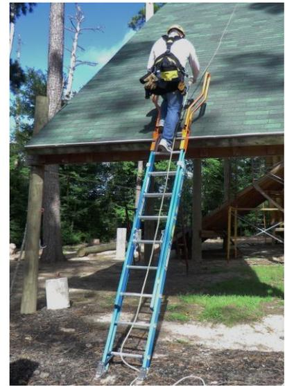
**Lateral Slippage** is the second most common cause of ladder related failure. It can take place with as little as 9 lbs of lateral pressure during the climber’s transition from ladder to roof or roof to ladder. Both kick-out and lateral slippage can be greatly reduced with the implementation of ladder stabilizing accessories.
